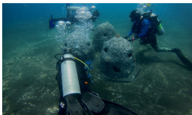
Gambar 5. Penanaman Terumbu Karang Hexadom
